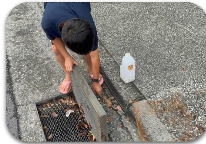
Setting Up Drainage Nets
